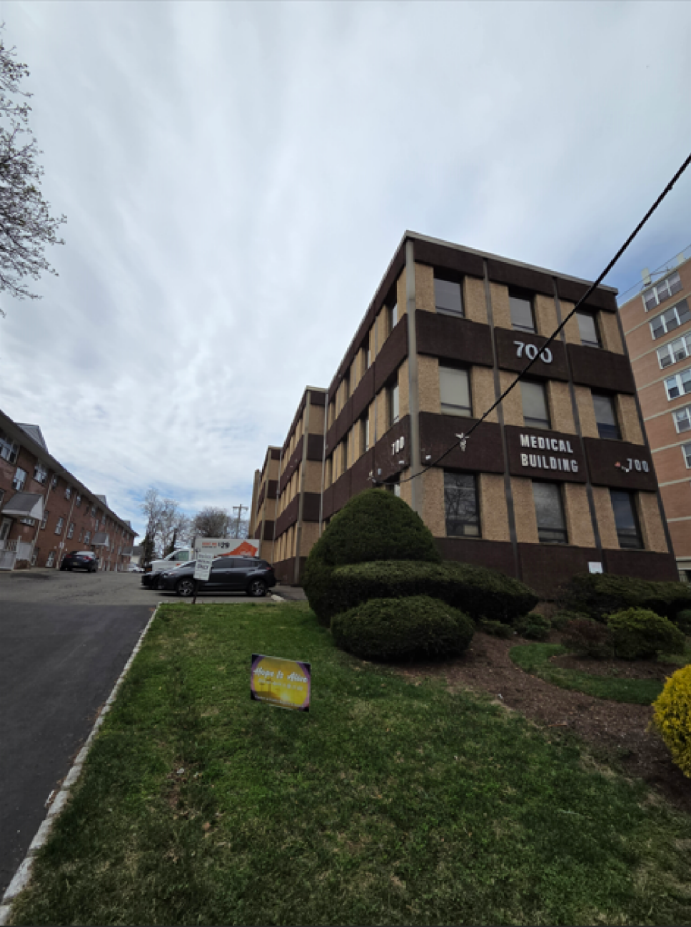
SITE PHOTO AS TAKEN ON 04.01.2026
