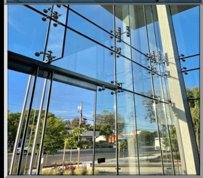
Structured Glass Lobby
