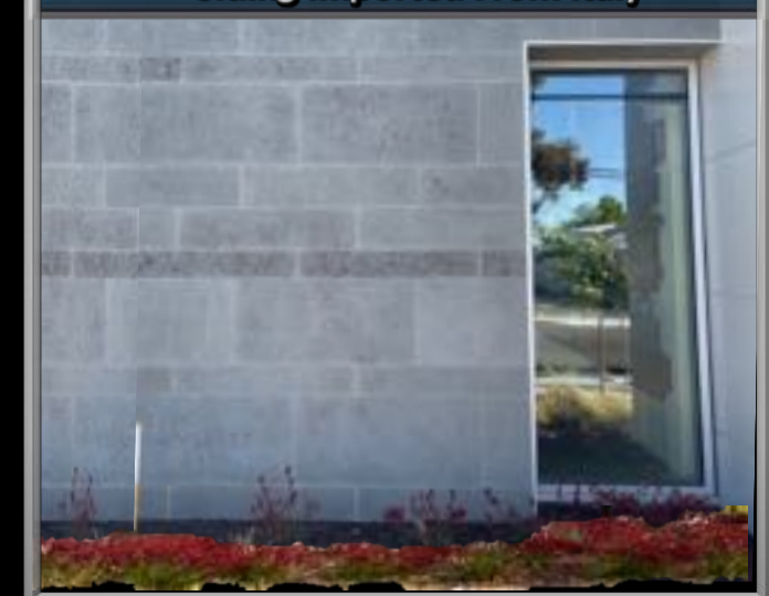
Lagos Azul Limestone Siding Imported From Italy
