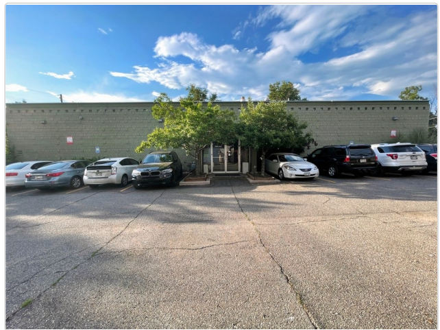
Building Exterior — 520 Cherokee St
