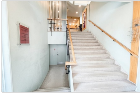
Building Entry & Staircase
