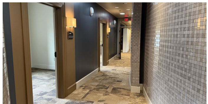
FINISHED CORRIDOR — OFFICE ENTRIES
