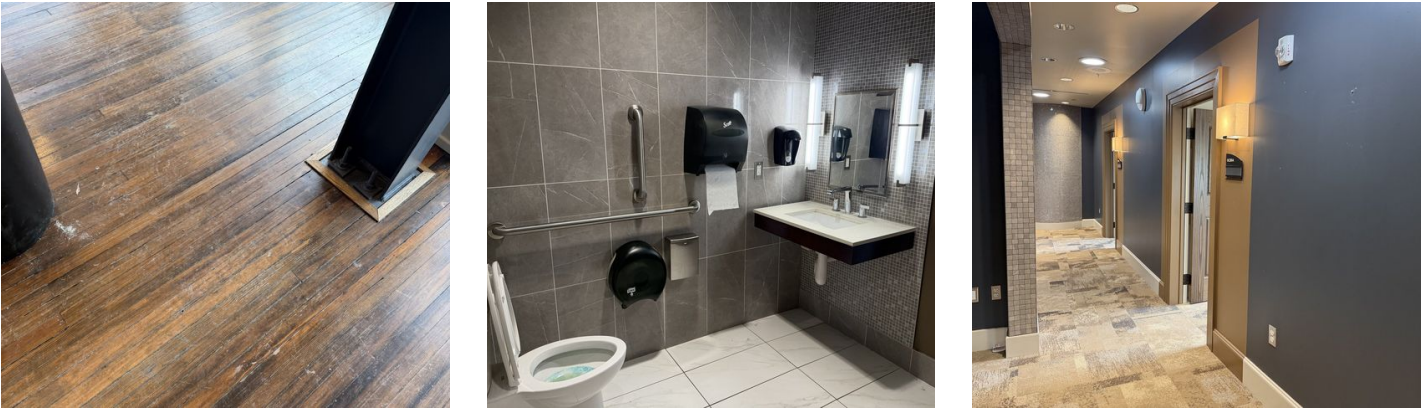
ORIGINAL HEART PINE FLOORING • RENOVATED RESTROOMS • THIRD FLOOR CORRIDOR
