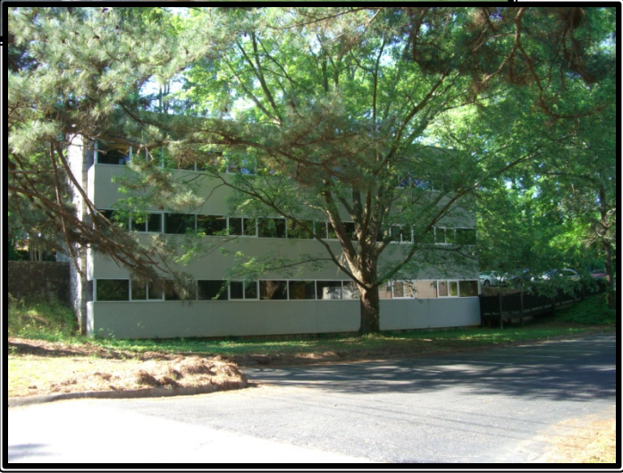
Exterior View of 3700 Longview Drive
