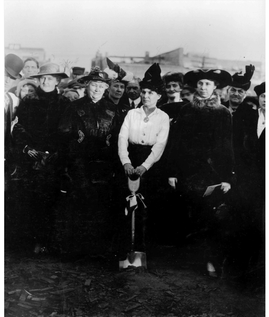
Breaking ground on the Carnegie Library, Sapulpa, circa 1918 (5420, Mat Duhr Collection, OHS).
