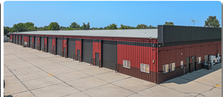
New tenant finishes included bathrooms, offices, monument sign, and exterior paint.
