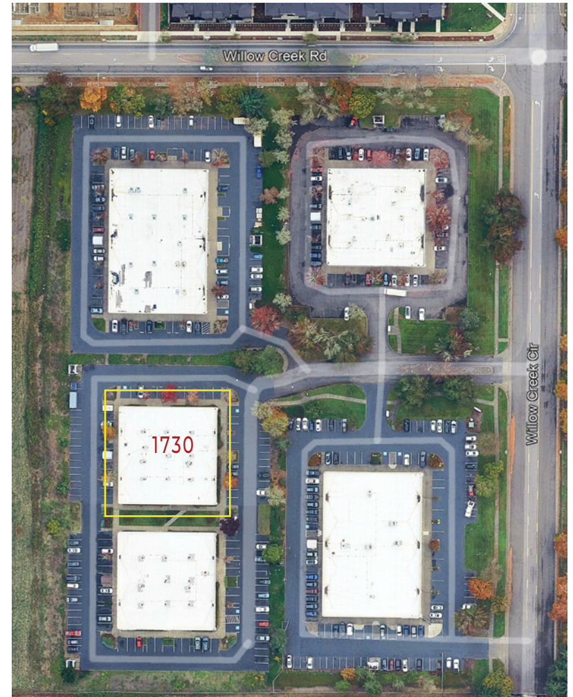
WESTEC BUSINESS PARK
