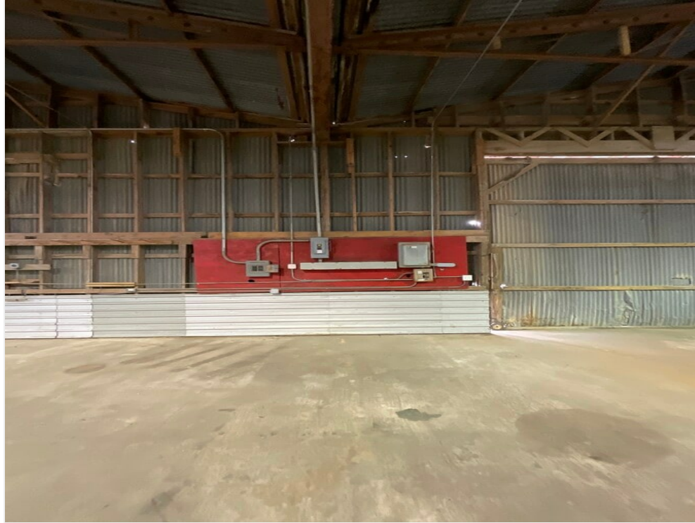
Warehouse Area of 3201 Texas Ave.
