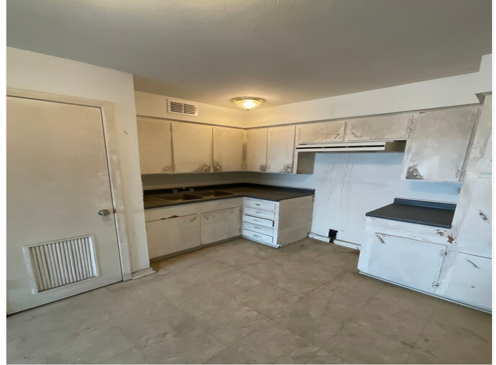
Apartment 2, Kitchen area
