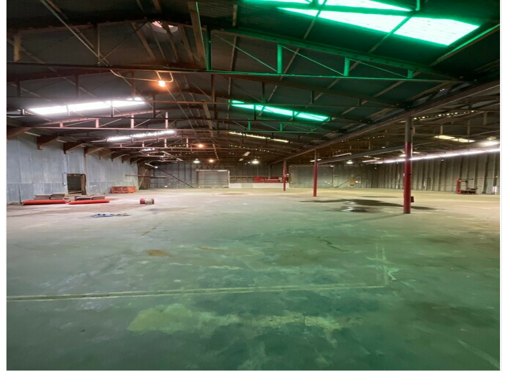
Warehouse Area of 3201 Texas Ave.
