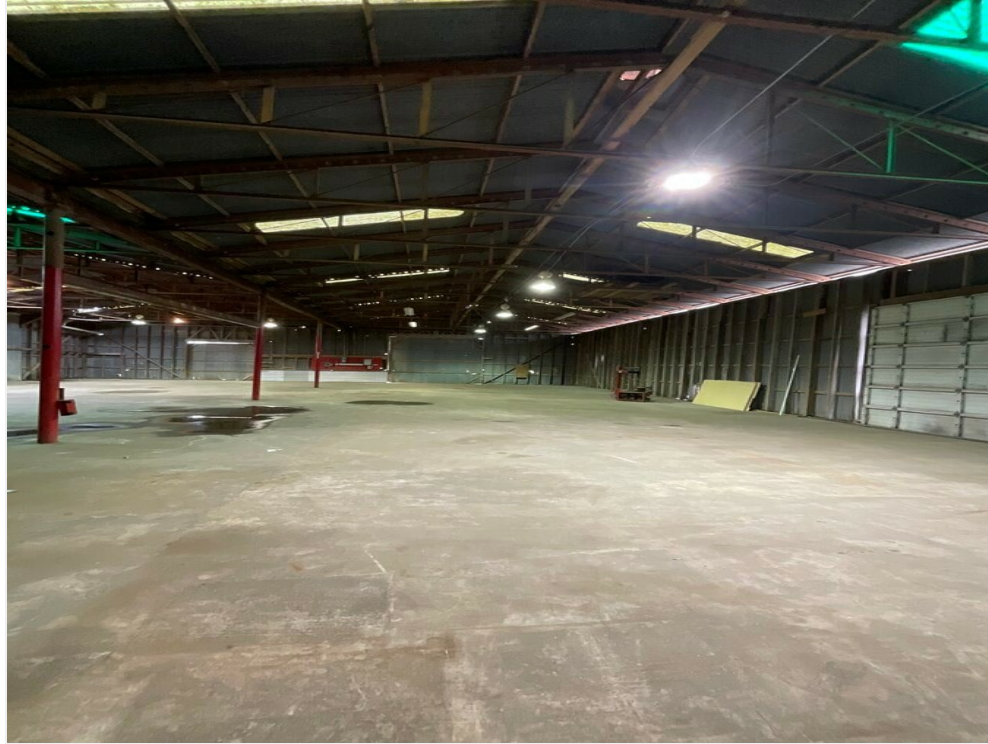
Warehouse Area of 3201 Texas Ave.
