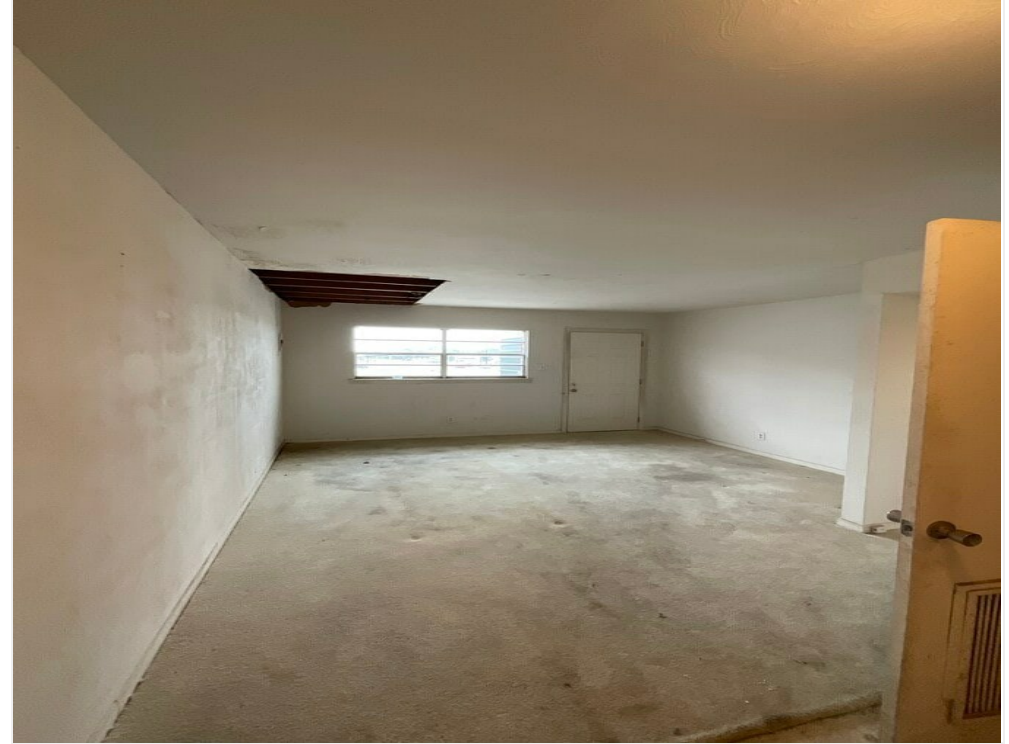
Warehouse Area of 3201 Texas Ave.
