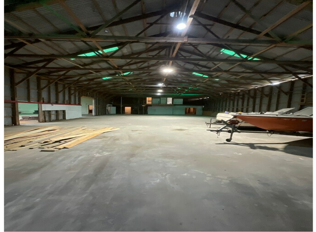
Warehouse Area of 3201 Texas Ave.
