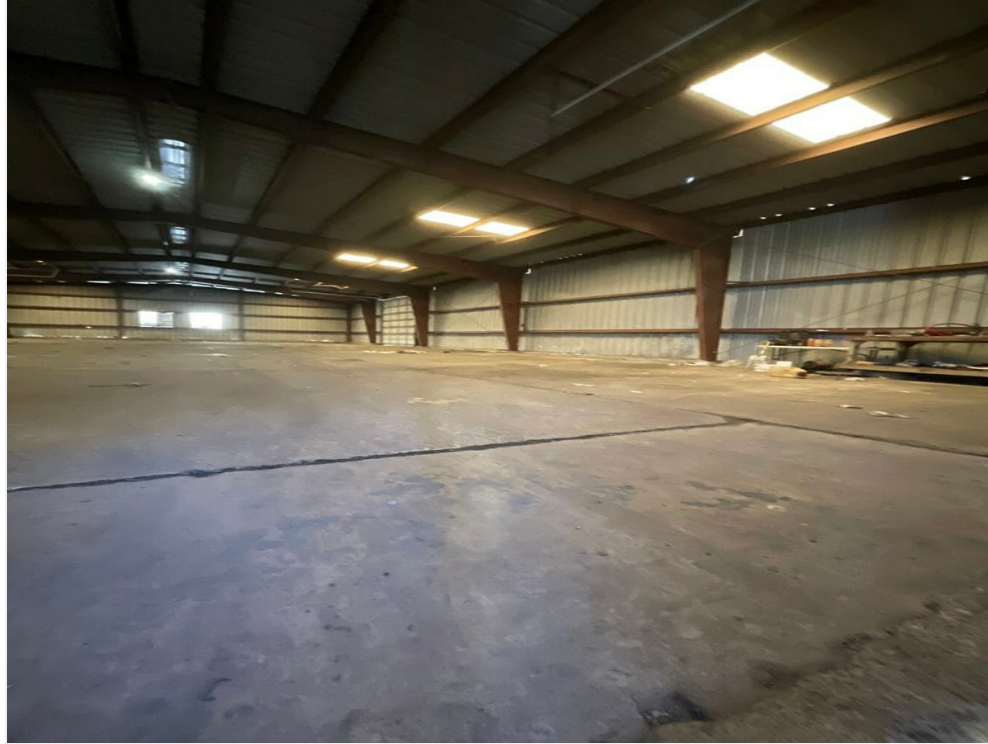
Inside the building at 2528 Jefferson
