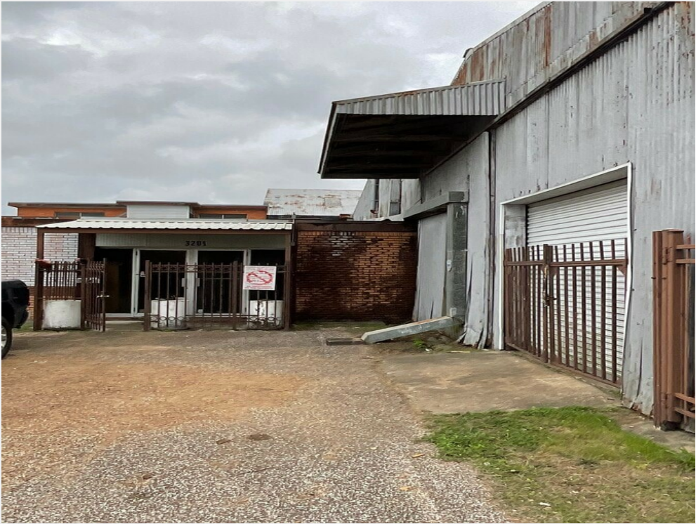
Front door of View of 3201 Texas Ave.
