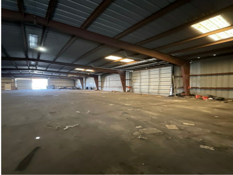
Inside the building at 2528 Jefferson
