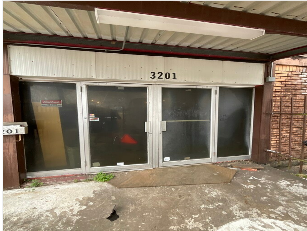
Front Door of View of 3201 Texas Ave.
