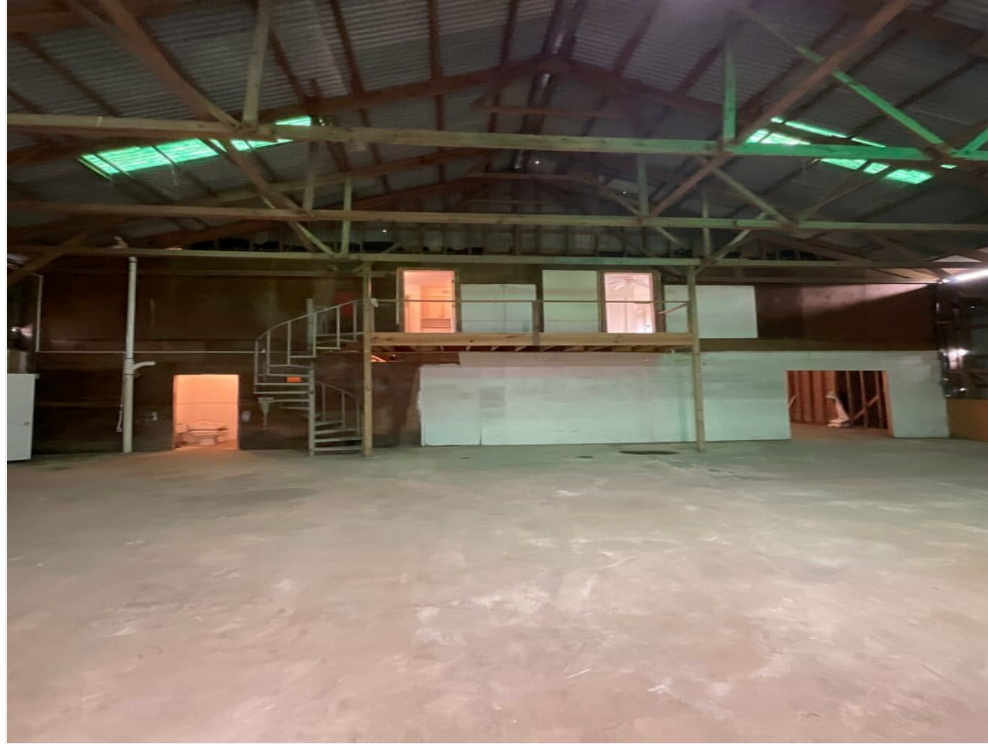
Warehouse Area of 3201 Texas Ave.
