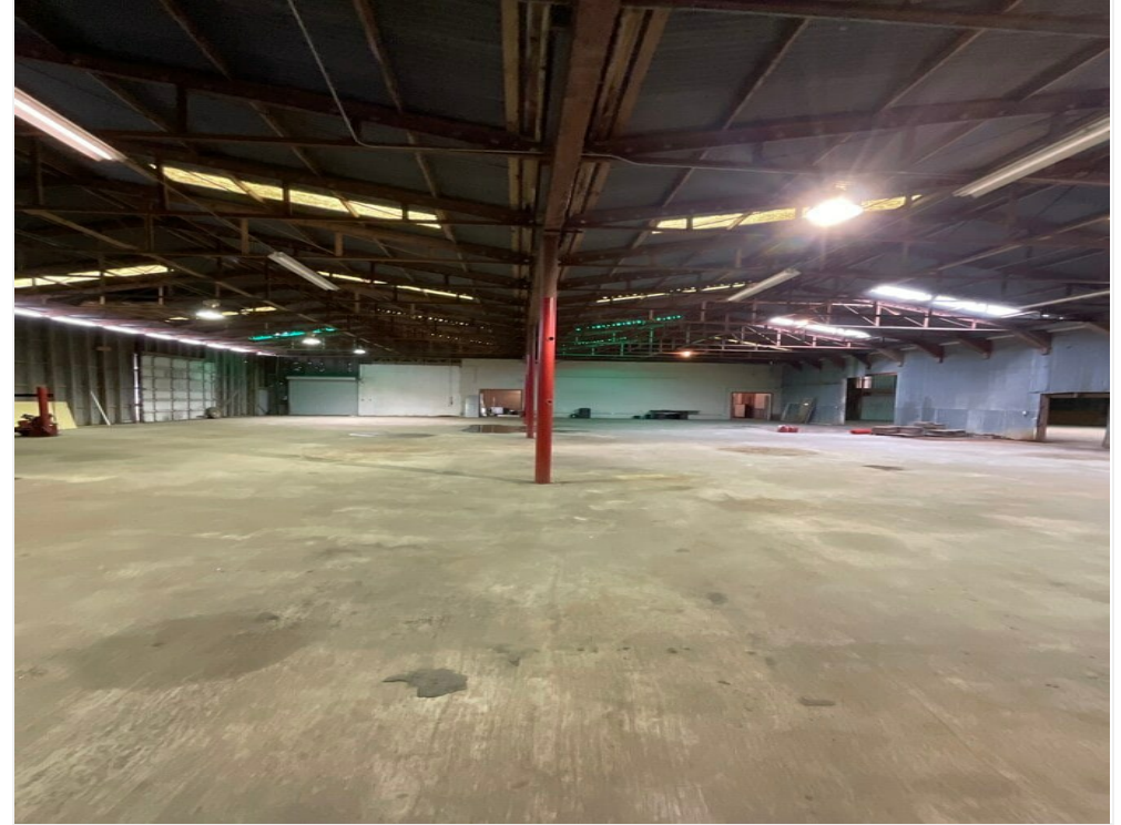
Warehouse Area of 3201 Texas Ave.
