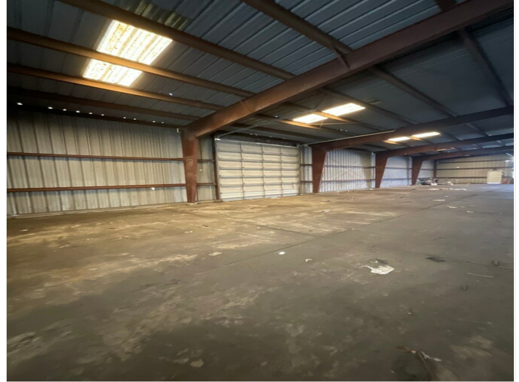
Inside the building at 2528 Jefferson
