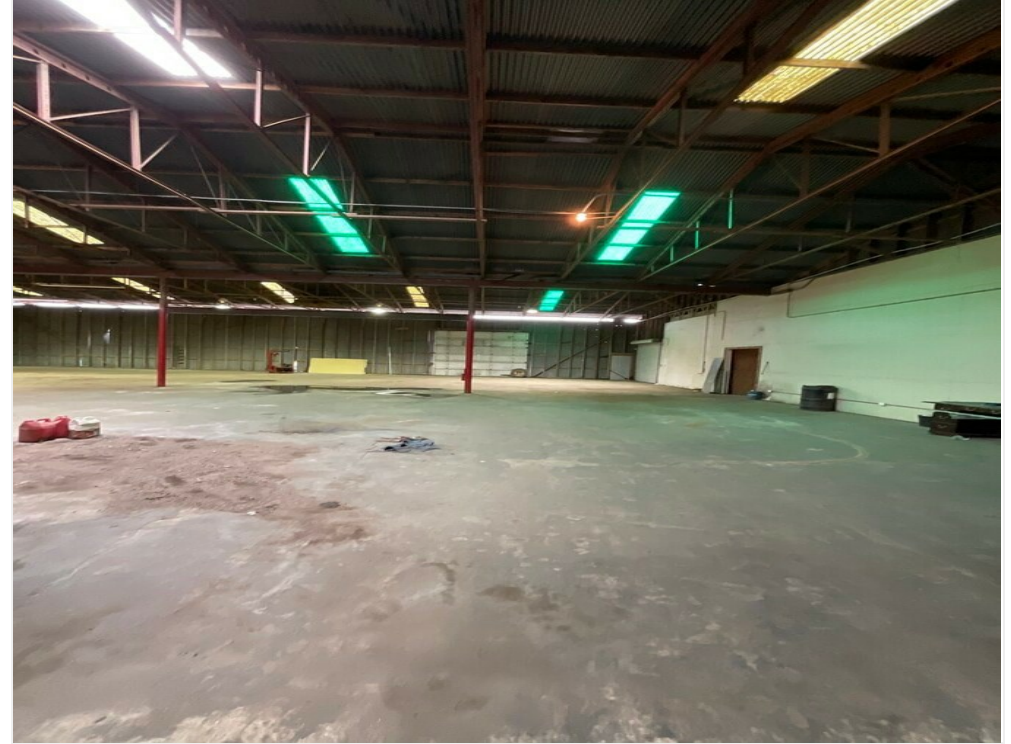
Warehouse Area of 3201 Texas Ave.
