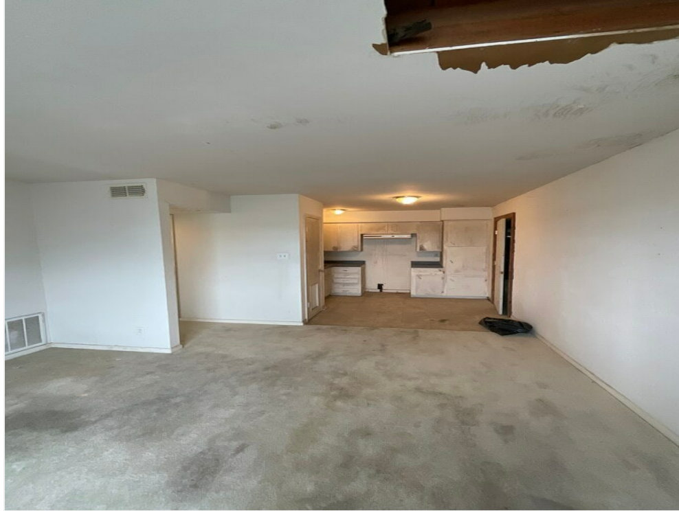
Apartment 1, living, dining, kitchen area
