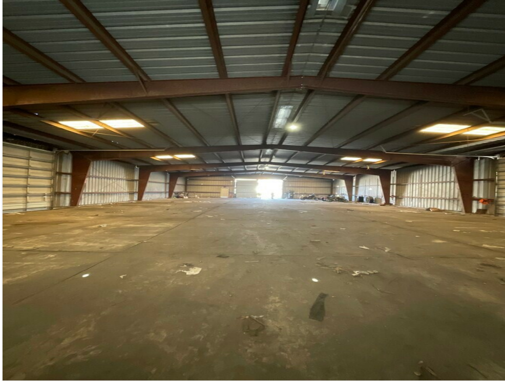
Inside the building at 2528 Jefferson
