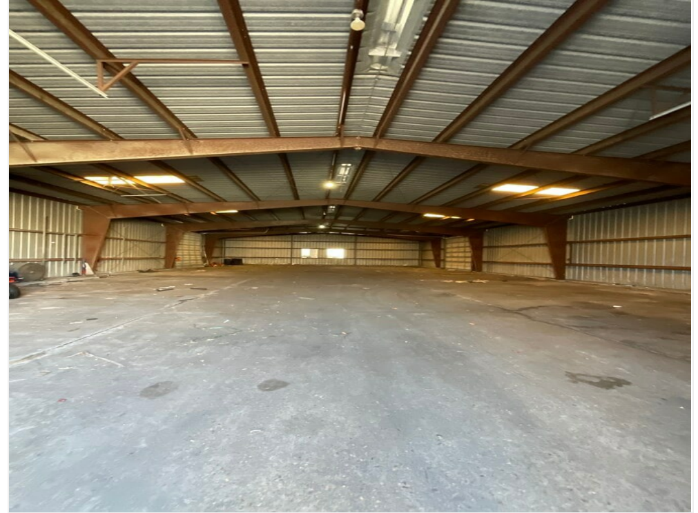
Inside the building at 2528 Jefferson
