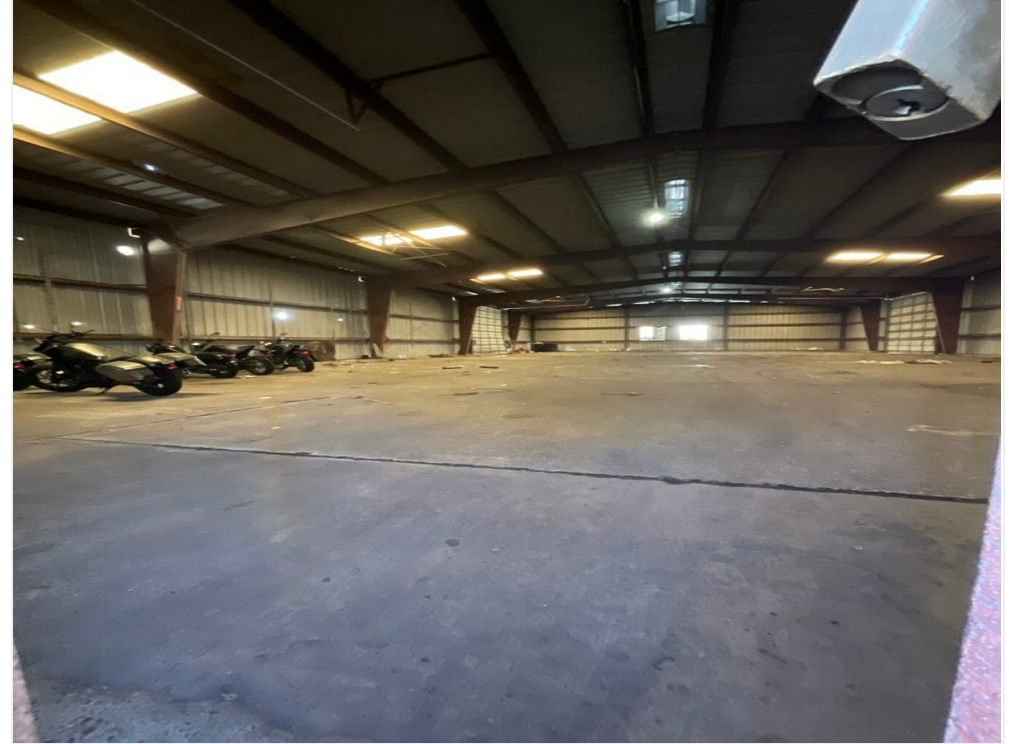
Inside the building at 2528 Jefferson
