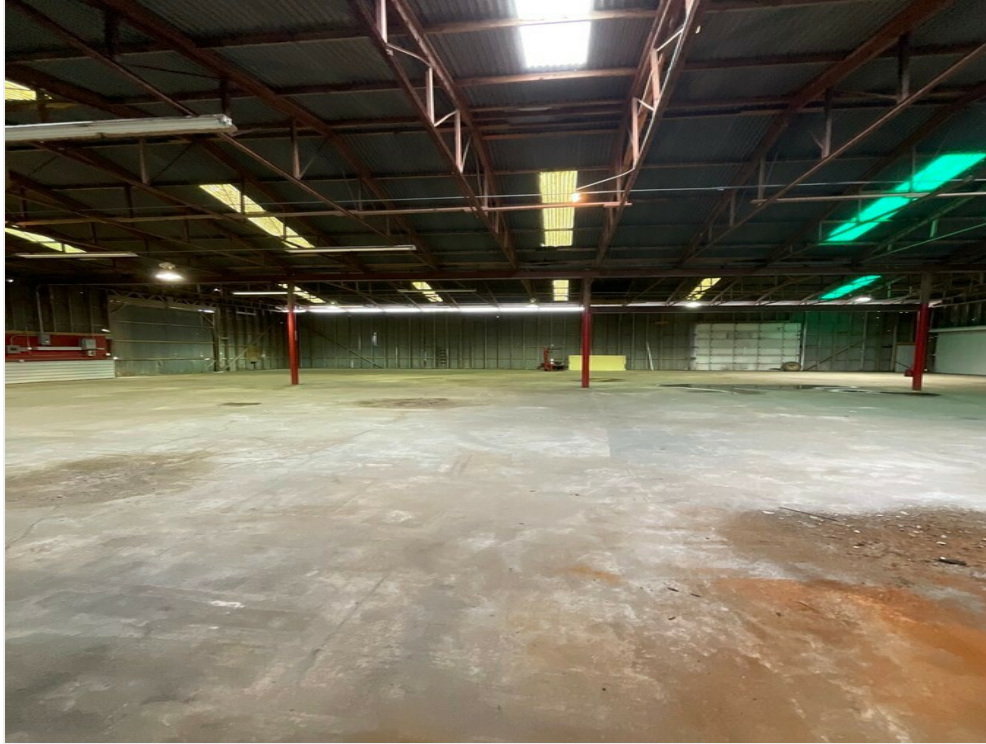
Warehouse Area of 3201 Texas Ave.
