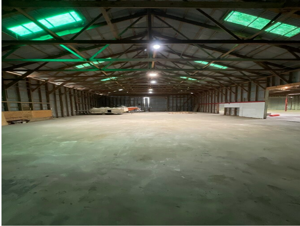
Warehouse Area of 3201 Texas Ave.
