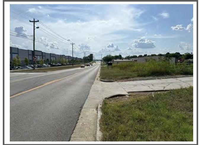
Site frontage along Beechcroft Road westbound
