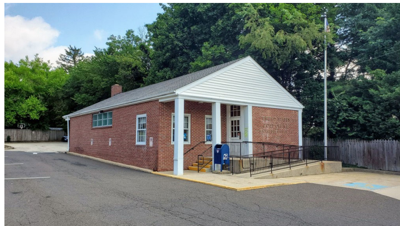
US POST OFFICE ACROSS STREET
