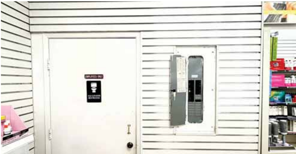
2842-#40 Story Road - Interior
