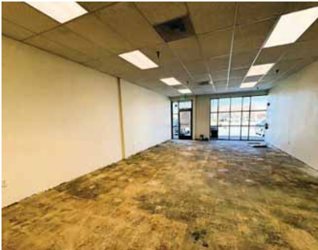
2842-#25 Story Road - Interior
