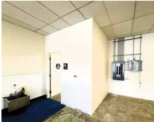
2842-#25 Story Road - Interior
