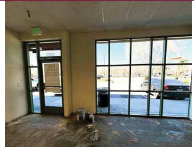
2842-#25 Story Road - Interior
