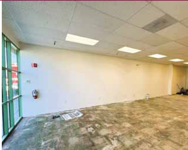
2842-#25 Story Road - Interior
