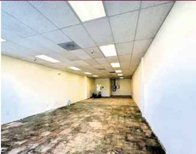
2842-#25 Story Road - Interior
