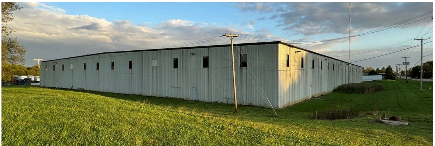
North Side of Building
