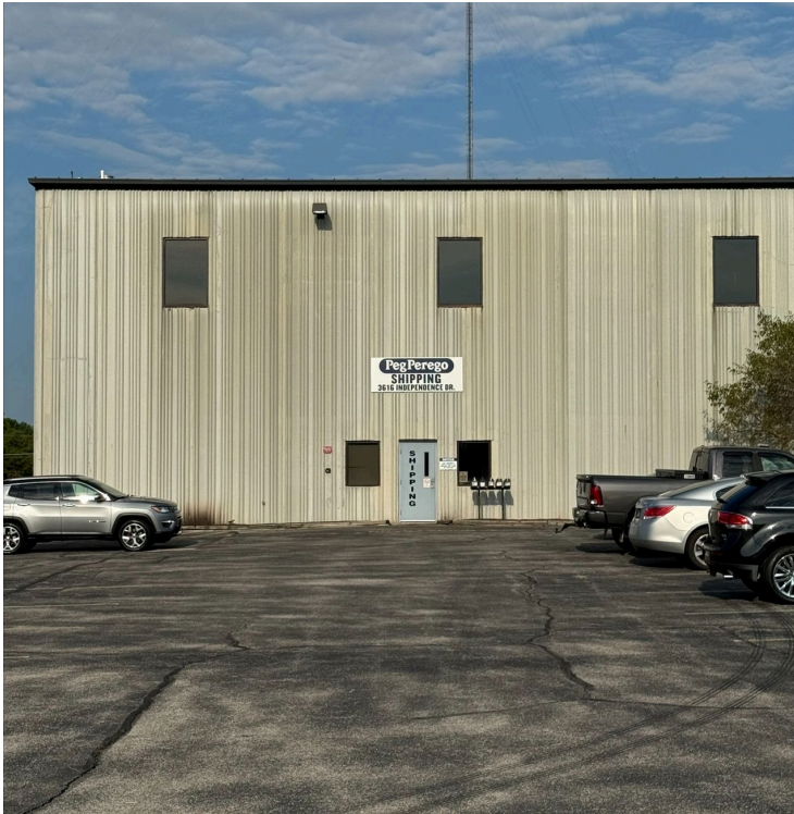
East Side of Building
