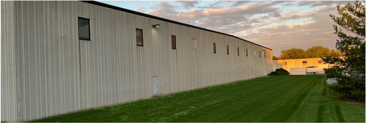
South Side of Building
