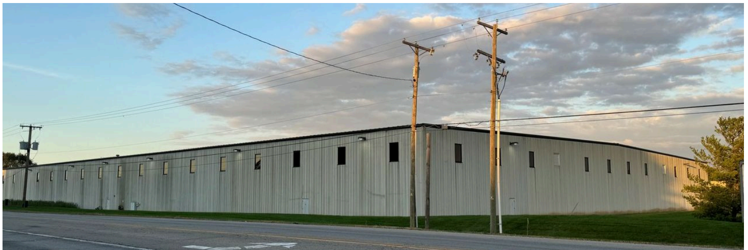
West Side of Building
