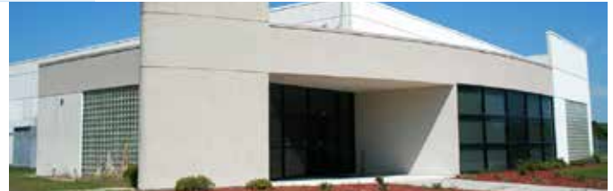
Exterior from southeast
