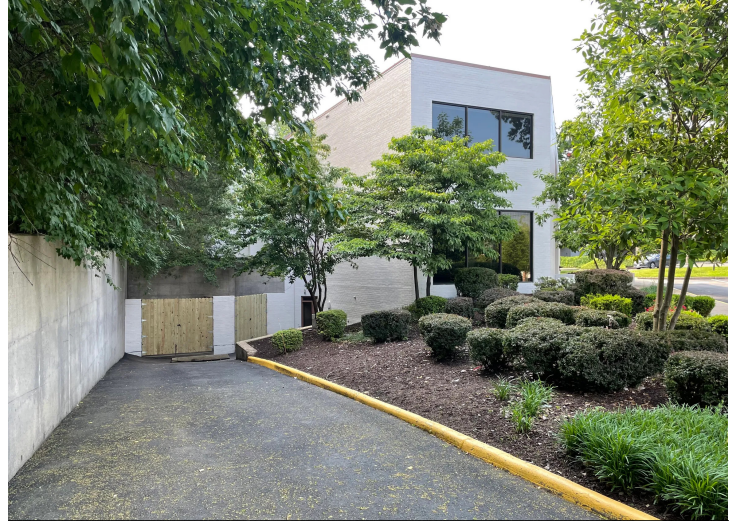
Front of Building and Loading Zone
