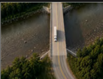
RUTHERFORD CREEK New Bridge — Site Connector
