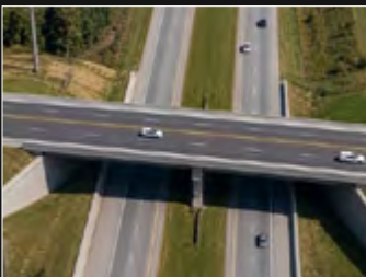
I-65 BRIDGE New Bridge — Master Connector
