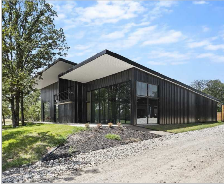
Central training building
