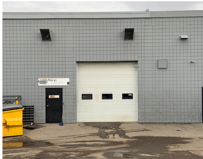
Rear Facing View – Loading
