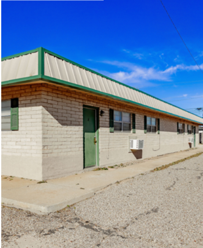
Tower Arms NORTH
