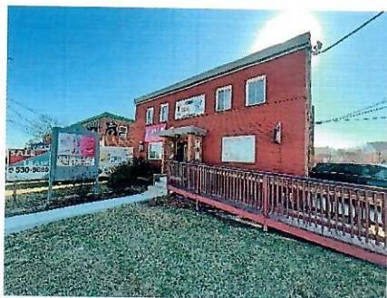
Exterior view of bldg. & sign
