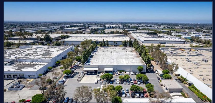
AERIAL SE · REAR YARD & LOADING
