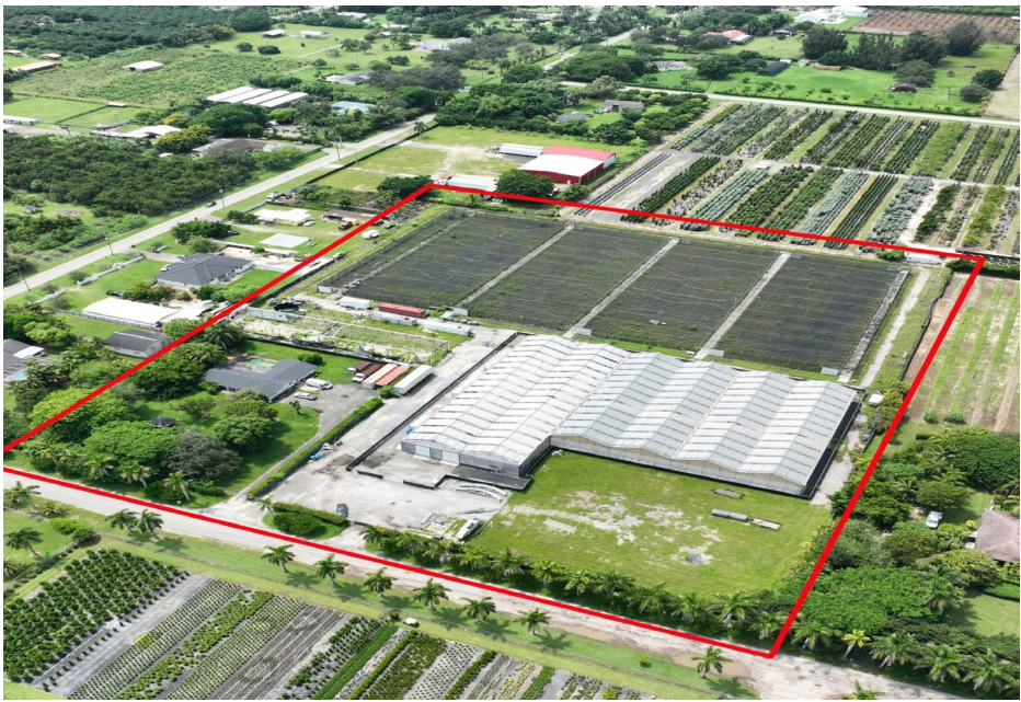
Aerial view — 6.10-acre nursery parcel outlined
