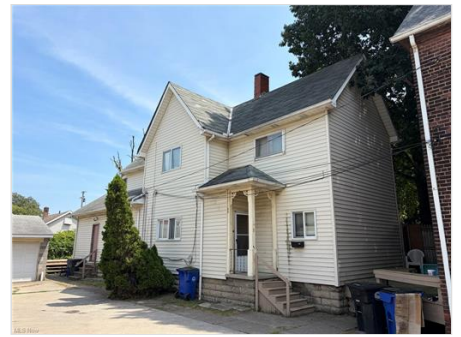
Back of Structure
