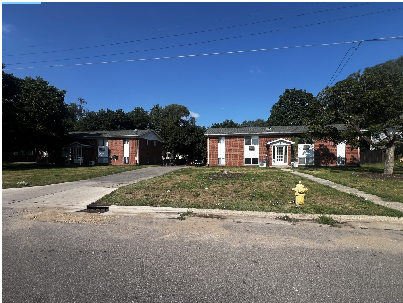
BOTH BUILDINGS • 3253 & 3275 CHARLESGATE
