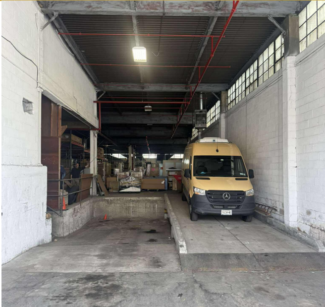
Loading Dock — Interior
