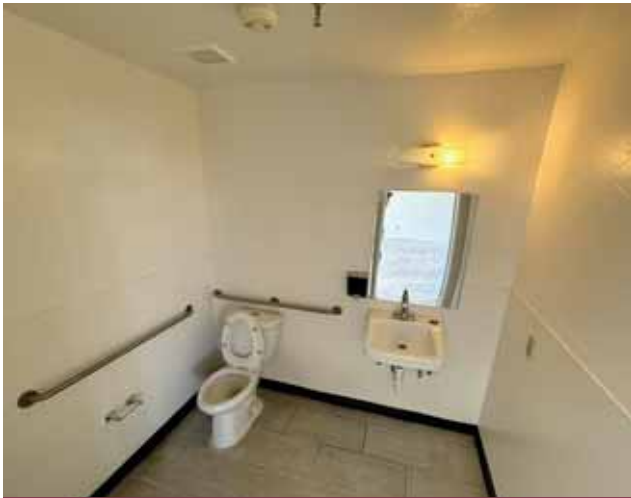
3093 McKee Road - ADA Restroom
