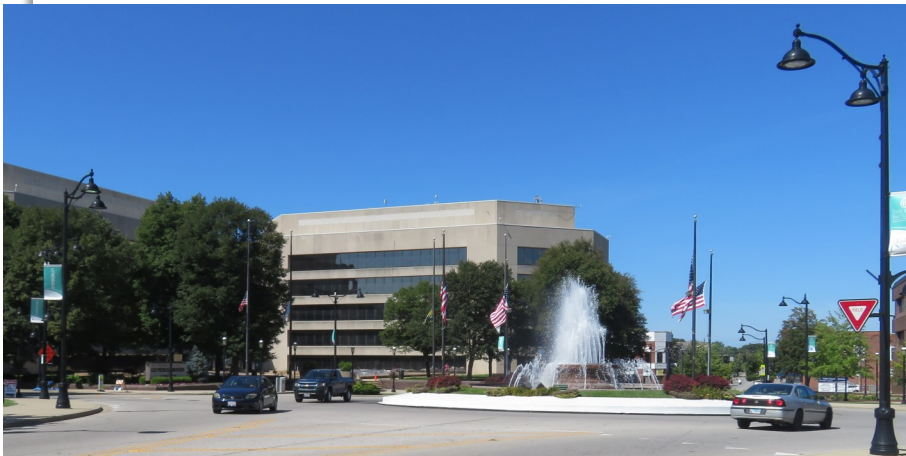
St. Clair County Court House on Belleville Public Square
