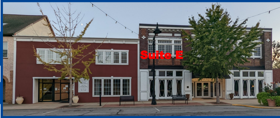
W. Main Street Entrance
