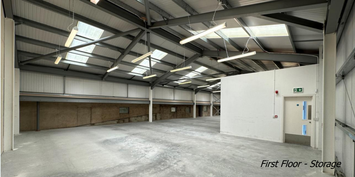
First Floor - Storage
