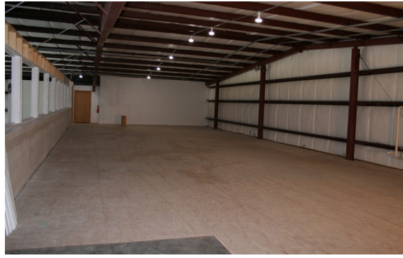
Loft area with led floodlights
