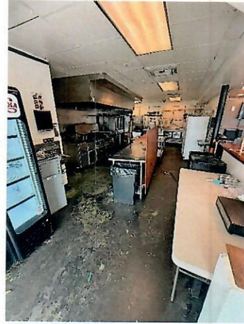
View of kitchen
