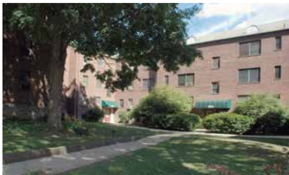
Community amenities include on-site laundry.
