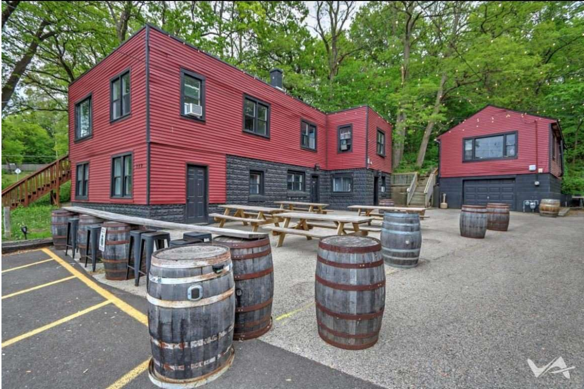
117 Nippersink — Rear elevation, courtyard seating, and detached structure
