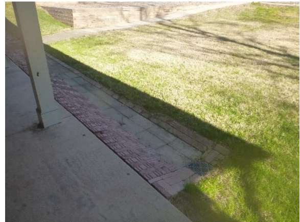
Area that drains into the existing Cistern, note landscape inlet to Cistern
