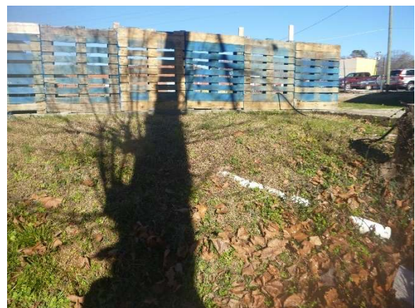
4" dia. Discharge pipe from existing Cistern
