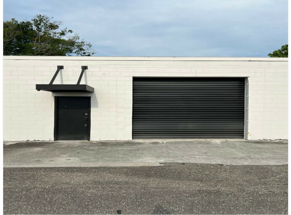
Unit A - Entry
