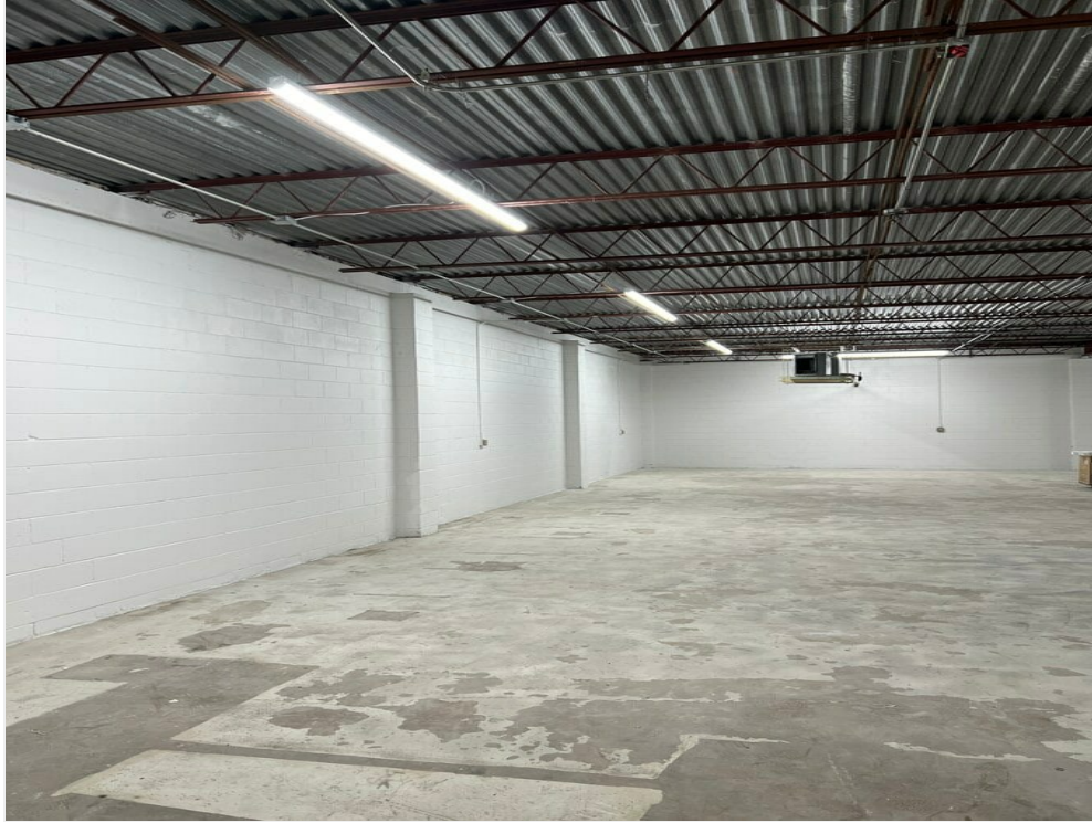
Interior - Unit B
