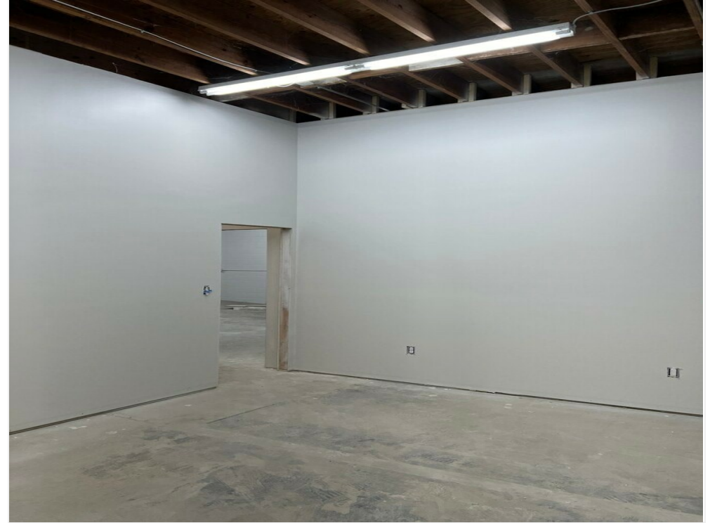
Front Office - Unit B
