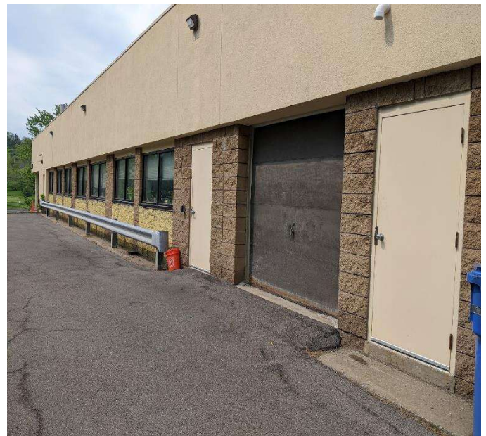
Exterior Overhead to Service & Trash Areas
