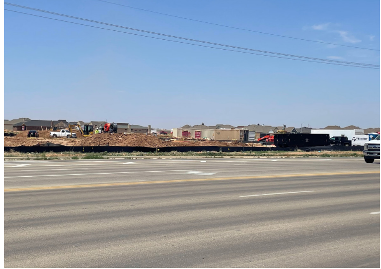
MCDONALD'S AND ALLIANCE CREDIT UNION UNDER CONSTRUCTION
