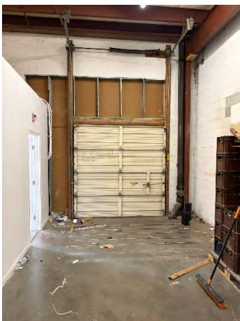
B10 View to Dock Door
