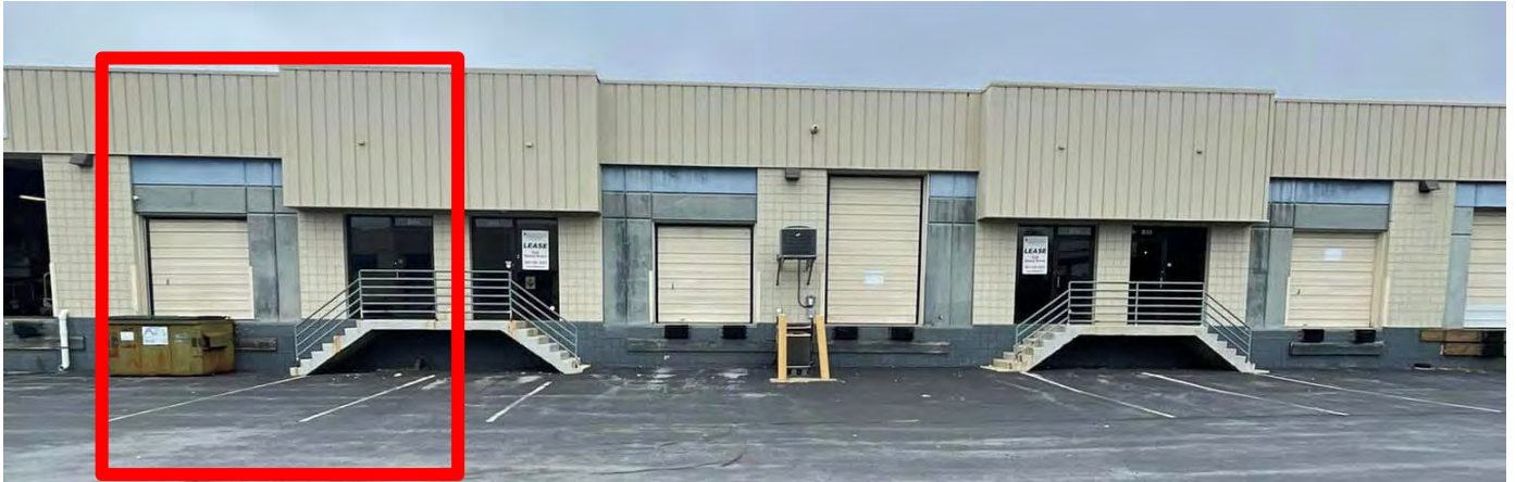
PEBC Suites B10 Exterior View – With Dock Door & Restroom
