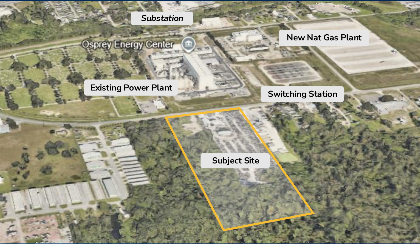
Subject site relative to adjacent generation, substation and switching infrastructure.
