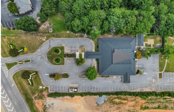
New roof / site overview
