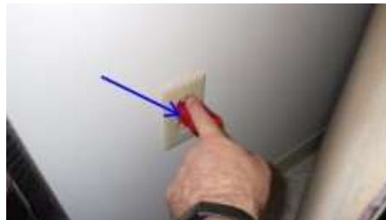
Install GFCI outlet.
