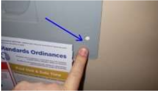
Install dead-front panel screw.
