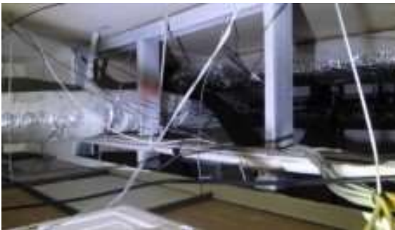
View of space above ceiling tiles.
