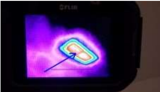
Heat verified at registers.
