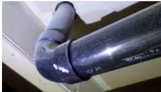
No signs of moisture noted above the tile.
