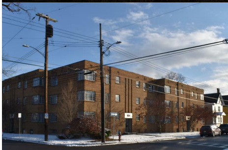
5. 162 CHAPIN STREET Binghamton, NY 13905
