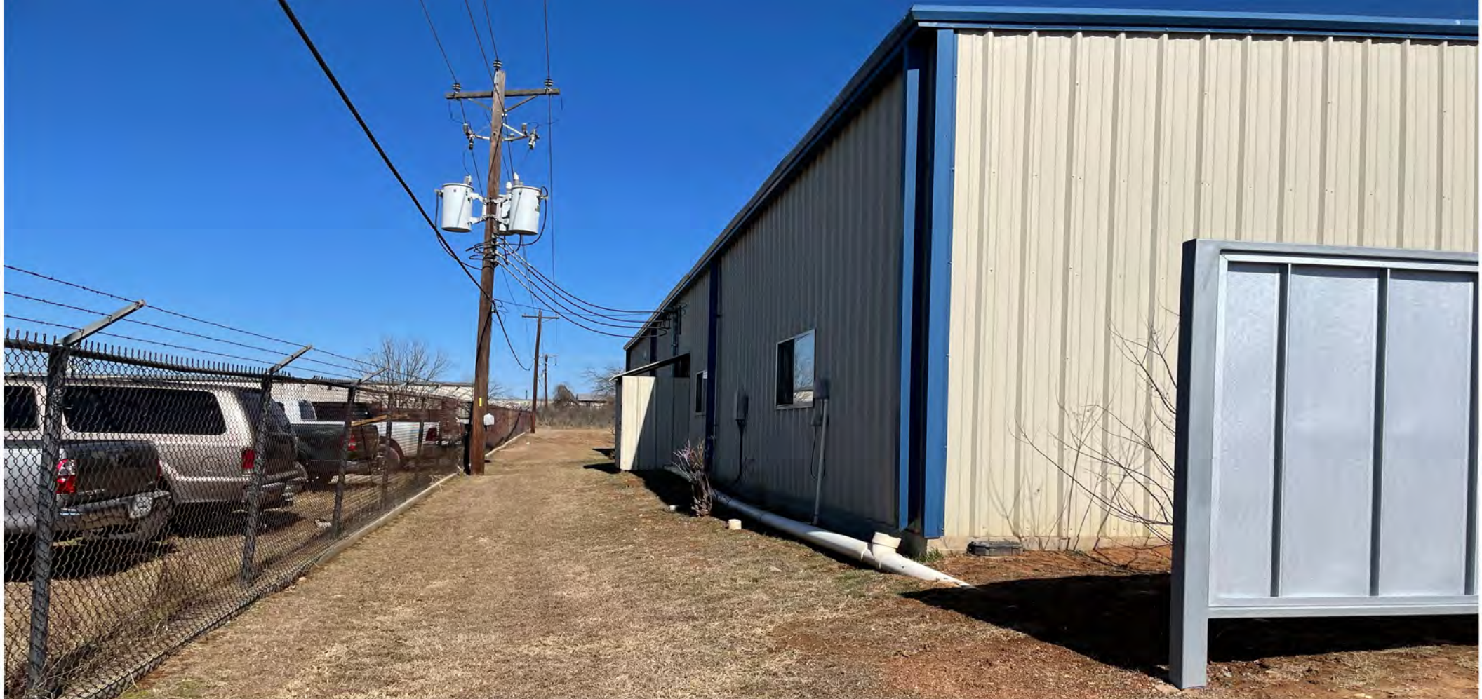
SOUTHWEST CORNER OF BLDG (LOOKING FROM FRONT - TO BACK OF PROPERTY)
