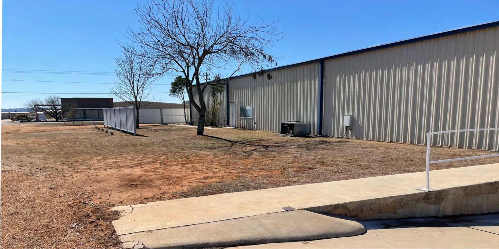
EAST SIDE OF BLDG LOOKING OUT TO FM 2093 FROM PARKING AND TRUCK WELL
