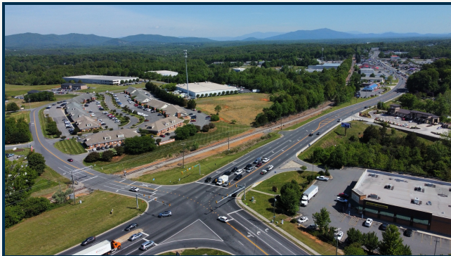
Signalized intersection at US Route 460 — direct site access and traffic corridor.
