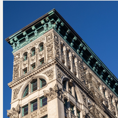
Cornice, 451 Broome St
