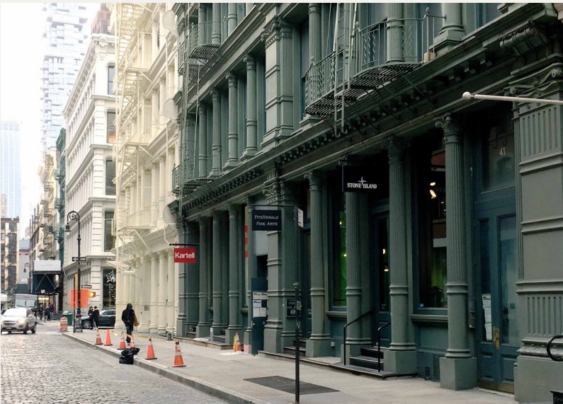
Cast-iron storefronts, SoHo
