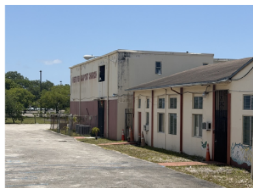
PAVED PARKING & SITE ACCESS
