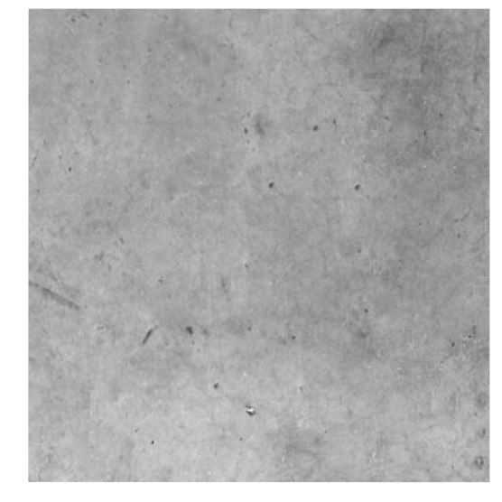
CAST IN PLACE CONCRETE
