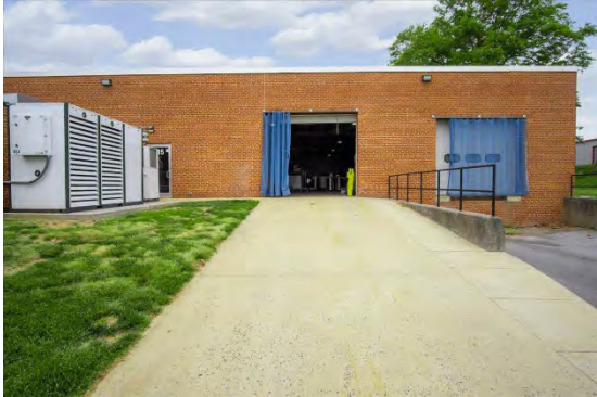
View of Drive In Door
