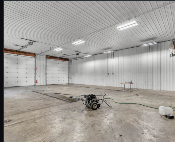
SERVICE BUILDING #3 28238 Markle Â· double bay interior
