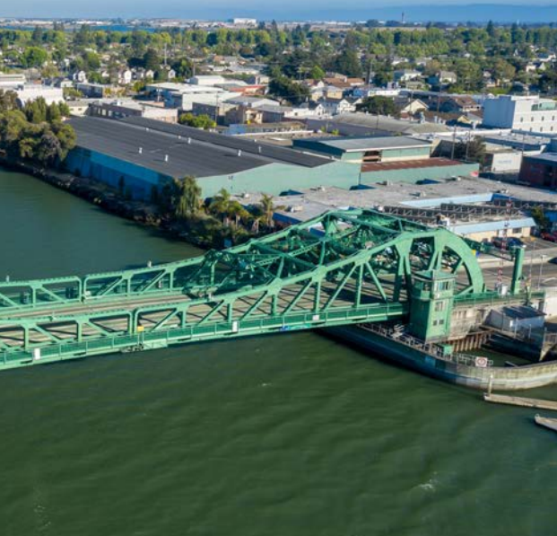
PARK STREET BRIDGE
