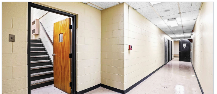
INTERIOR CIRCULATION & STAIR ACCESS
